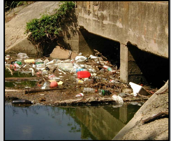
Trash and debris
