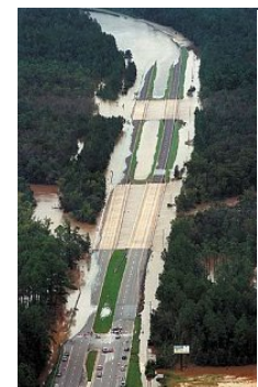
An aerial photograph (left) of State Road 85 looking south shows the extent of the flooding around the Shoal River Bridge, which was closed in 1998.
