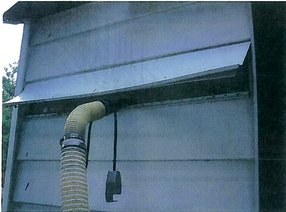
Installation of Blown-in Insulation
